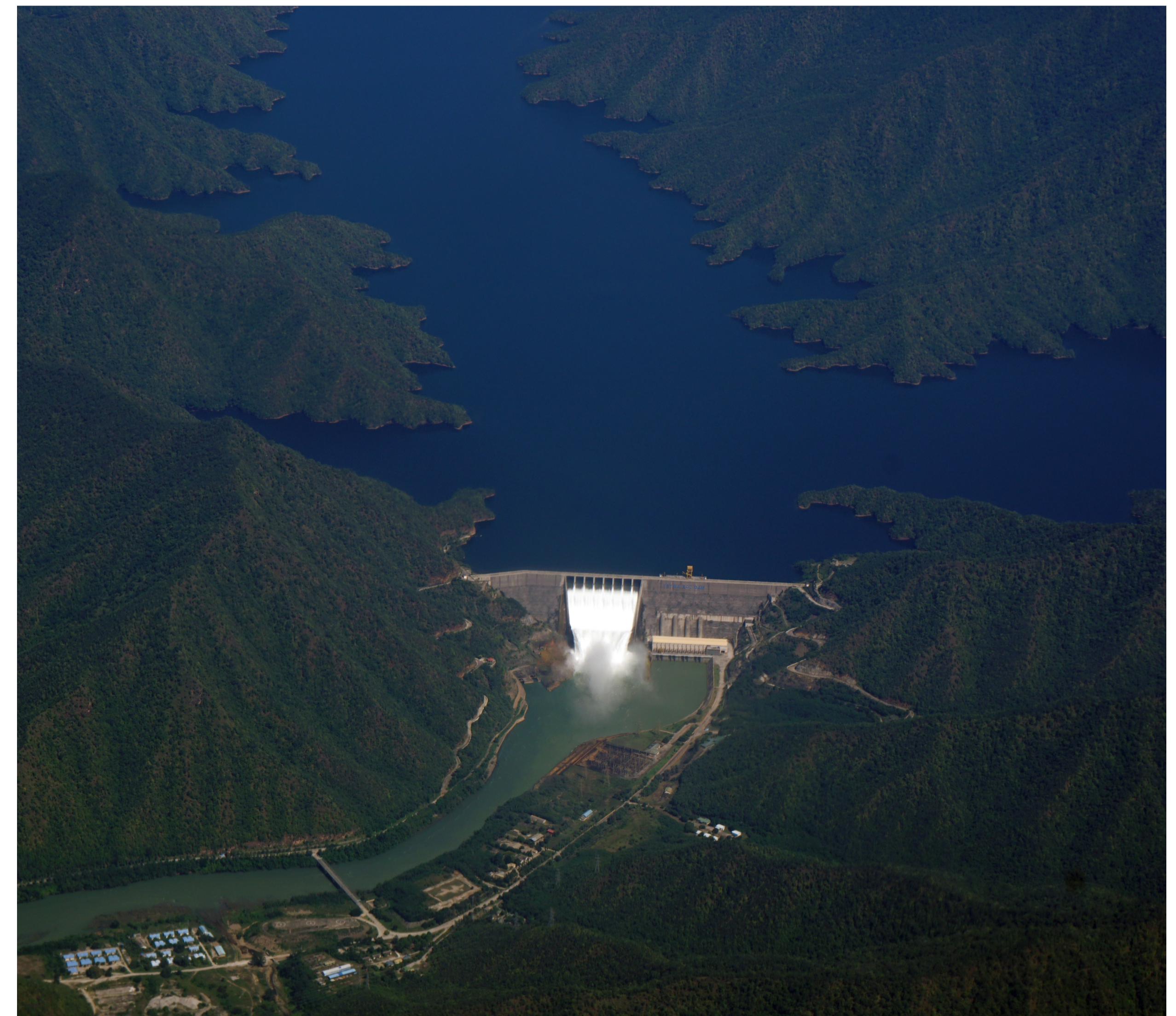
Hydroelectric Dam in Myanmar/ Shutterstock
